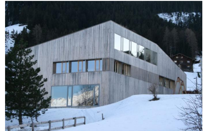
Offices, Germany, Architect Hermann Kaufmann
