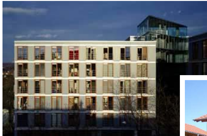
Student residence refurbishment – Neue Bourse, University of Wuppertal, Germany
